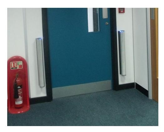
Designed to integrate seamlessly with Access Control, CCTV and whole building management systems. By receiving information from your Access Control system, Door Detective products know how many people to admit and in which direction of travel. Any unexpected movements are instantly met with an audible and visual alarm and signals are passed to your Access Control or CCTV system to acknowledge that alarm condition has occurred.
