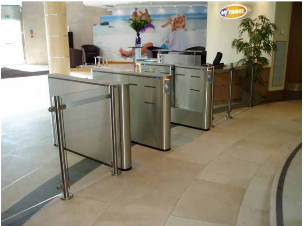
Fastlane Glassgate installed on site, original image available on request.
